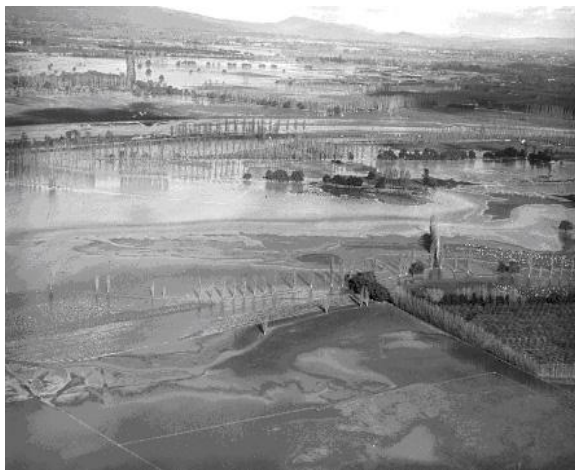
Flood 1935 (before stopbanks)
