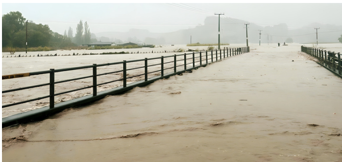
Ohiwia Bridge in Omahu during the Cyclone
