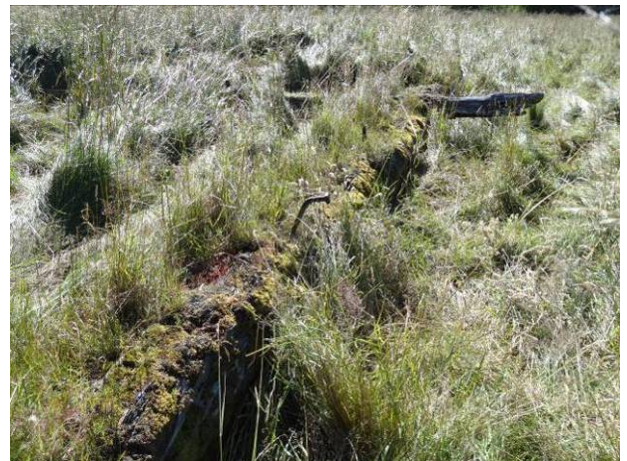
Figure 29. Wooden bearer with iron bolt and cross beam (part of the Mill floor)
