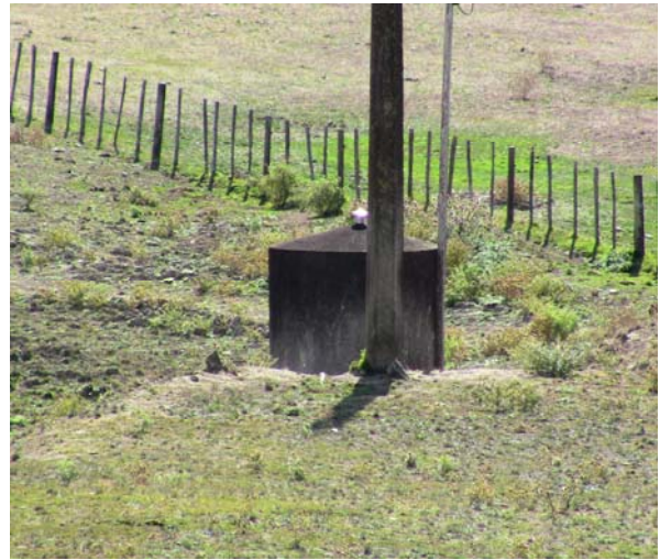
Pump Shed marks Looking Glass
